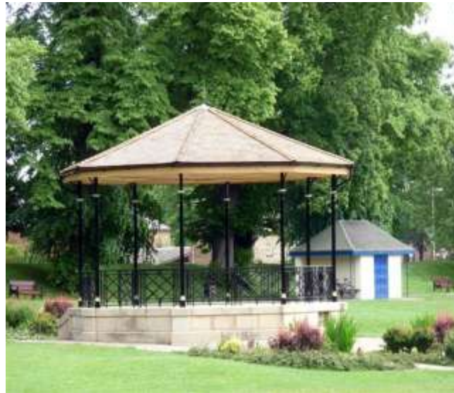
Newly refurbished bandstand May 2010
